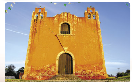
A typical colonial church in Santa Elena
